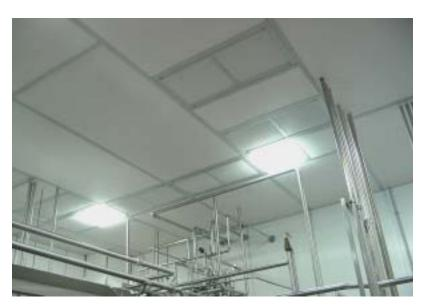
Aluminum extrusions have been specially anodized to withstand chemicals and acids associated with dairy operations. Once installed this ceiling system meets and exceeds American National Standard A58.1-1982 for accessible ceilings.
