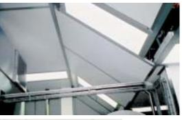
Gay Lea. "In addition, the walls were required to support window, doors and conveyor openings. All wall joints had to be positively sealed as the room will be under positive
